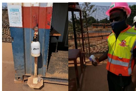
Figure 16: The WBHO construction site
