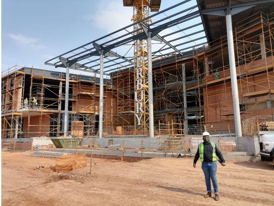
Figure 15: WBHO Pretoria construction site
