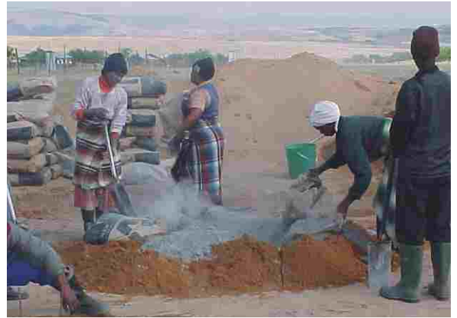
Manufacturing cement blocks for reservoir and pumphouse walls
