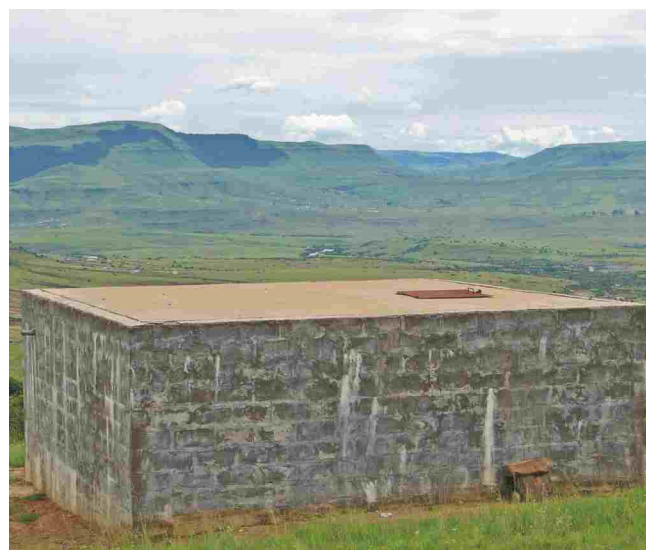
Finished reservoir in operation
