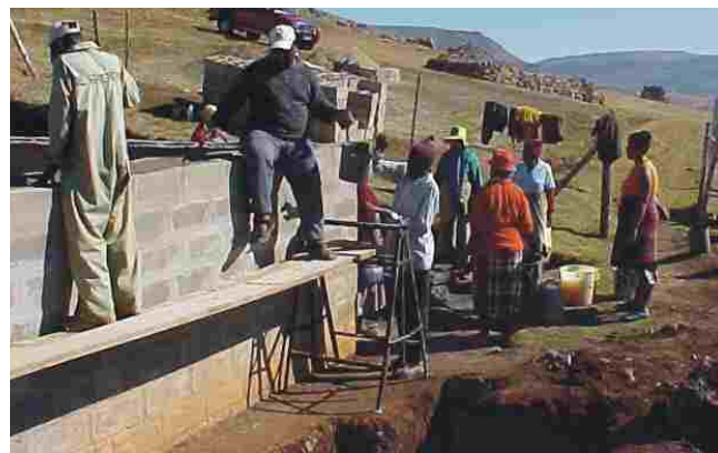
Building the reservoir
