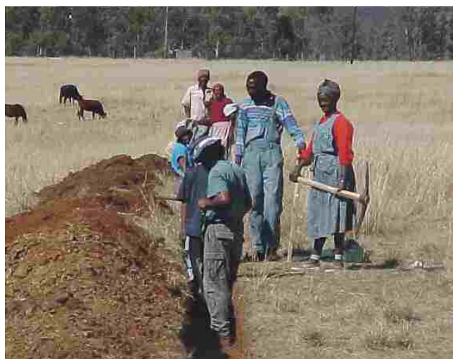
Community members digging pipe trenches
