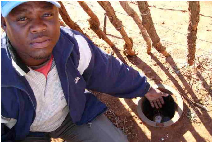
Newly installed water meter in Thomo Village
