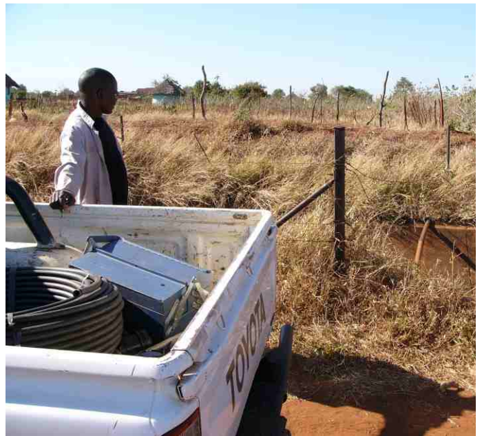
Municipal maintenance team inspect illegal connection
