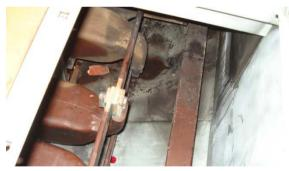
MANY PREVIOUS FAULTS – MOSTLY FROM CABLE TERMINATION FAULTS PANEL NOT BEEN CLEANED ADEQUATELY LEADING SECONDARY FAULTS
