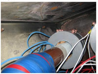
PARTIAL DISCHARGE DETECTED ON VT AND REPLACEMENT CT'S NOT INSTALLED CORRECTLY OEM DESIGN PROBLEM AND POOR WORKMANSHIP
