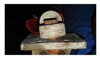
LOOSE CONNECTION CAUSED EXCESSIVE HEAT TERMINATION REPLACED
