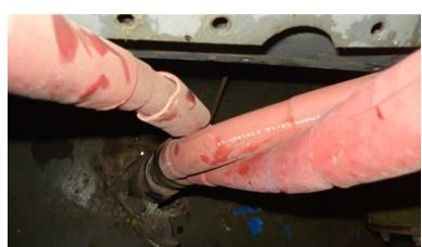
COMPOUND FILLED TERMINATION REPLACED WITH HEAT SHRINK INDEQUATE CLEARENCES AND CORE CROSSED
