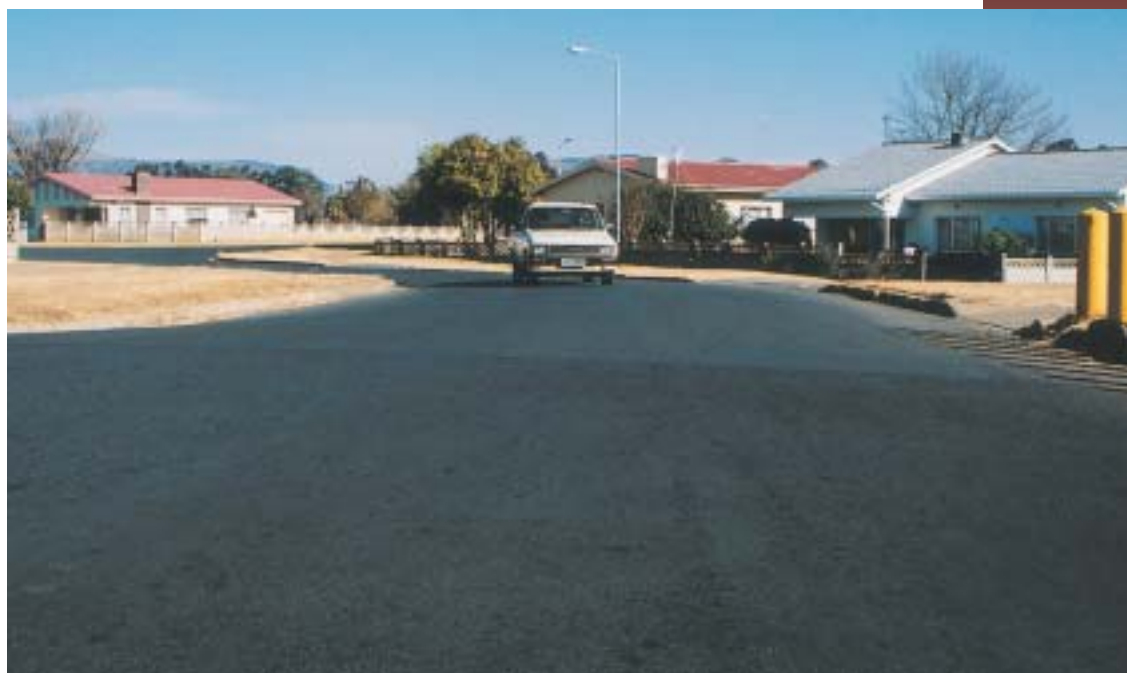
The Endumeni Municipality infrastructure development programme, KwaZulu-Natal
