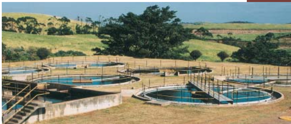
Dolphin Coast water and sanitation infrastructure, KwaZulu-Natal
