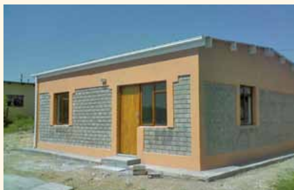
A completed house on Ngozi Street constructed from Hydraform interlocking low-cement blocks.
