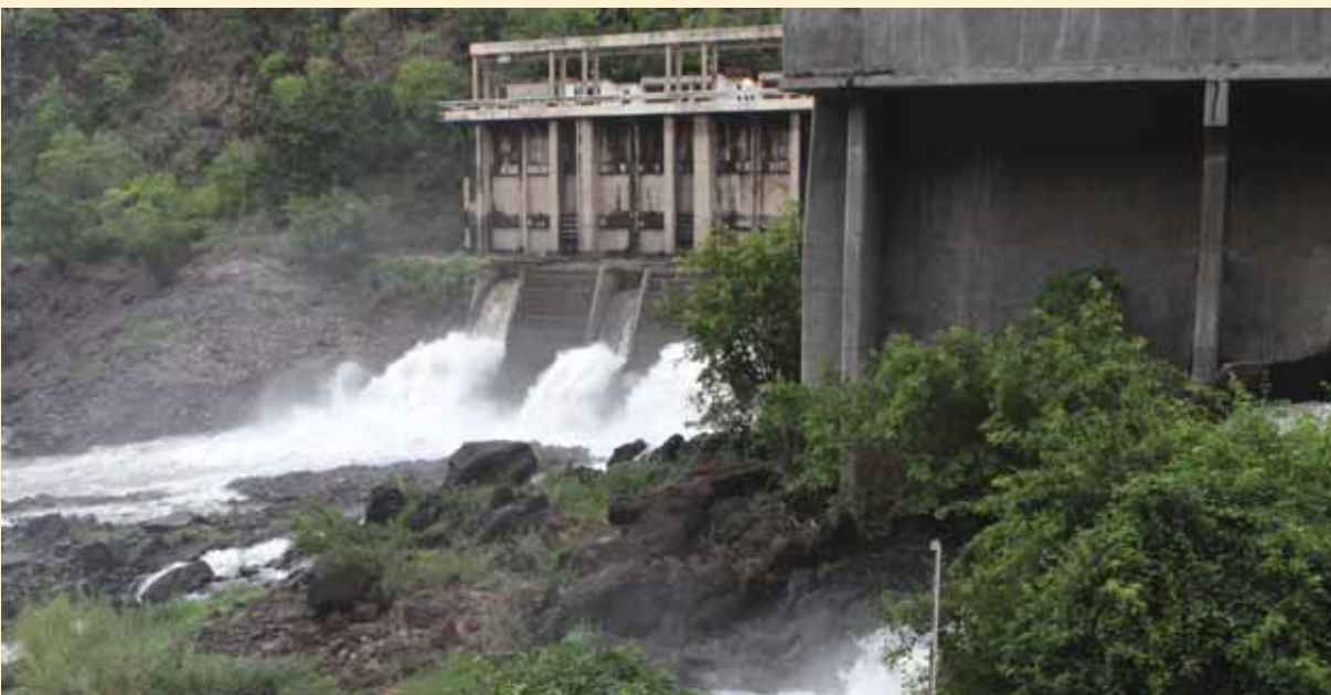
The DBSA was a member of an international team advising ZESCO on the development of two power stations in Zambia.
