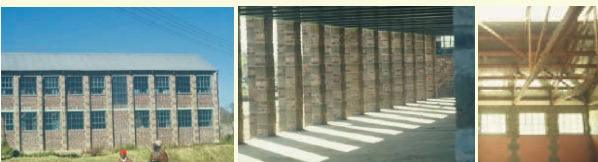
Urban sites utilising passive solar heating with Trombe walls
