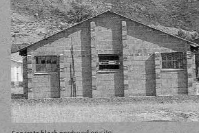
Concrete block produced on site.
