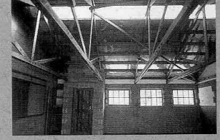
Classroom showing roof structure and infill walls.
