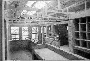
Library resource rooms.
