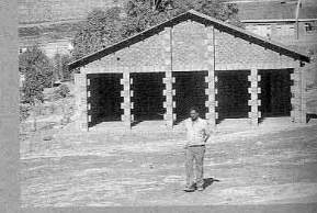
Open-framed classroom before infill.
