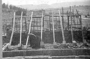
Window and door infill fits exactly between columns.
