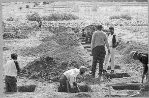
Setting out of the pad foundation.
