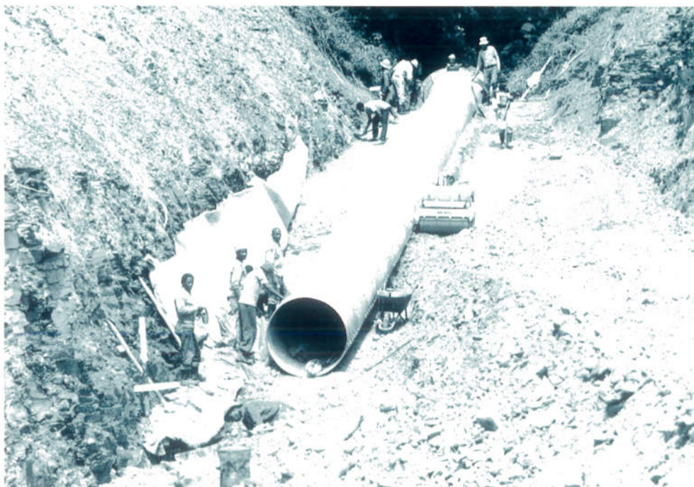
Construction work on stormwater drainage for the upgrading of road R61 between Lusikisiki and Port St Johns in Transkei. Apart from considering the economic merits of infrastructure development projects, the Bank also gives thorough attention to providing the maximum scope for labour-intensive construction approaches, appropriate designs and the use of local goods and materials.
