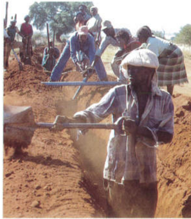
Villagers from Mabeskraal line trenches with soft soil to accommodate the trunk mains that will bring water to their village in arid northern Bophuthatswana.
