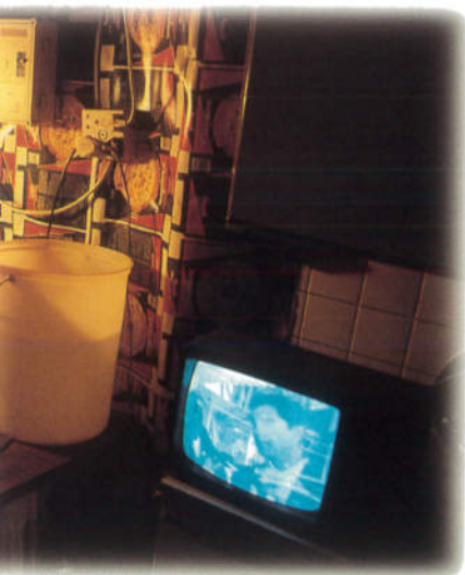
Transitional Electricity Distributor Programme: Mpumalanga
