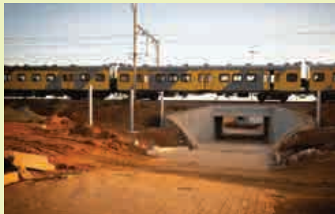
Underpass crossing bridge at the end of phase one
