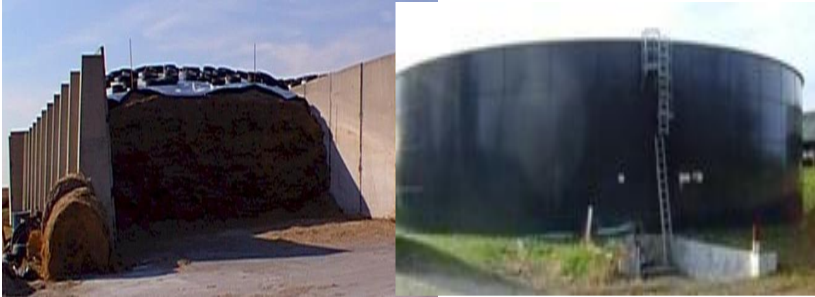
Figure 6-7 Bunker silo made of concrete and covered by plastic foils (left) and Slurry tank (right)
