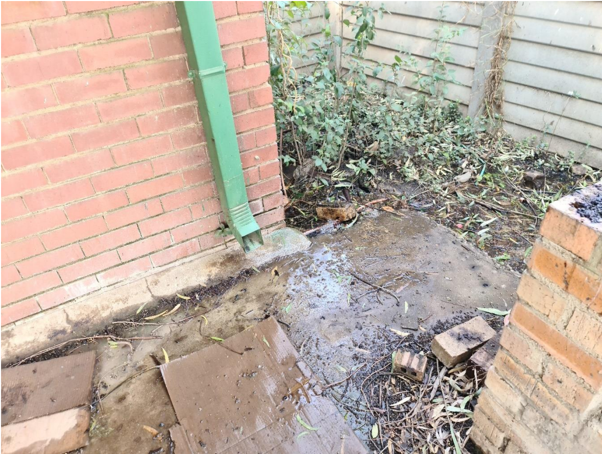
Figure 18: Outside water supply pipe leak.
