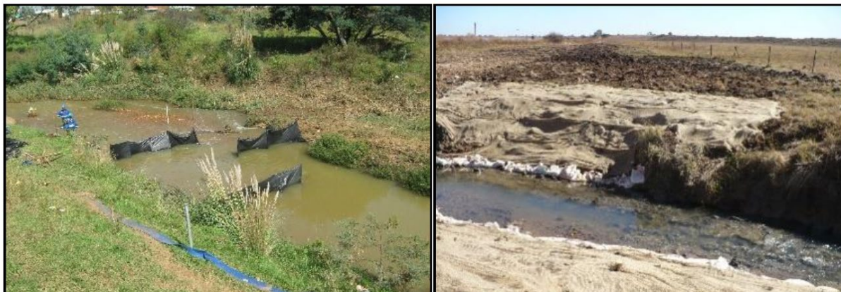
Figure 4.1: Examples of sediment/silt traps to be used during the construction phase, to limit additional sediment from entering downstream reach of the floodplain wetland; during (Left) instream activities; (Right) activities directly adjacent to the freshwater ecosystem.
