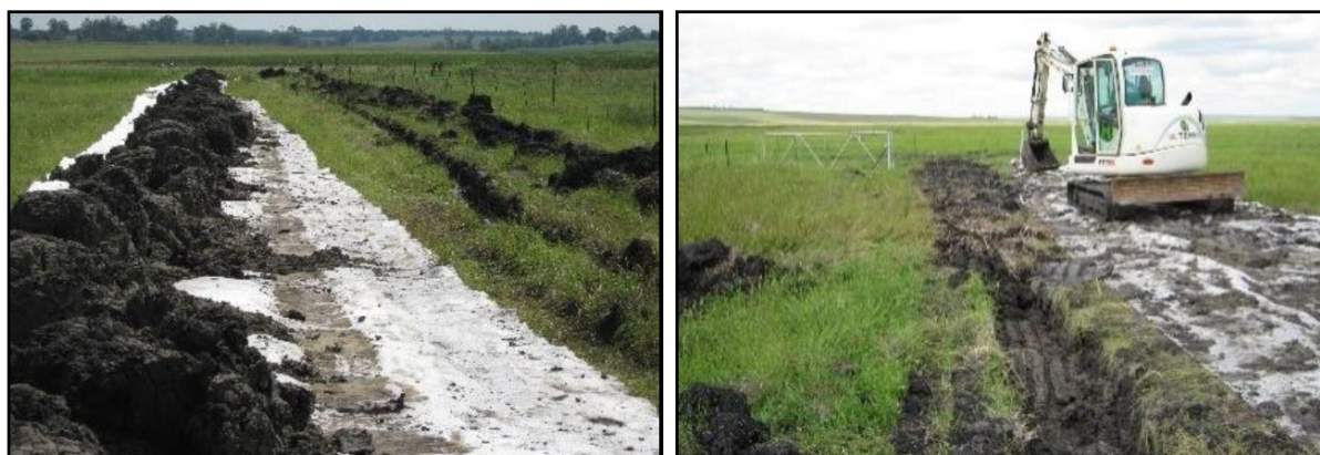
Figure 4.2: (Left) Excavation for pipe trenching with stockpiles alongside; (Right) Backfilling of the trench with the construction vehicle remaining on one side of the disturbance footprint. Note the use of bog mats to limit impact on wetland soils.
