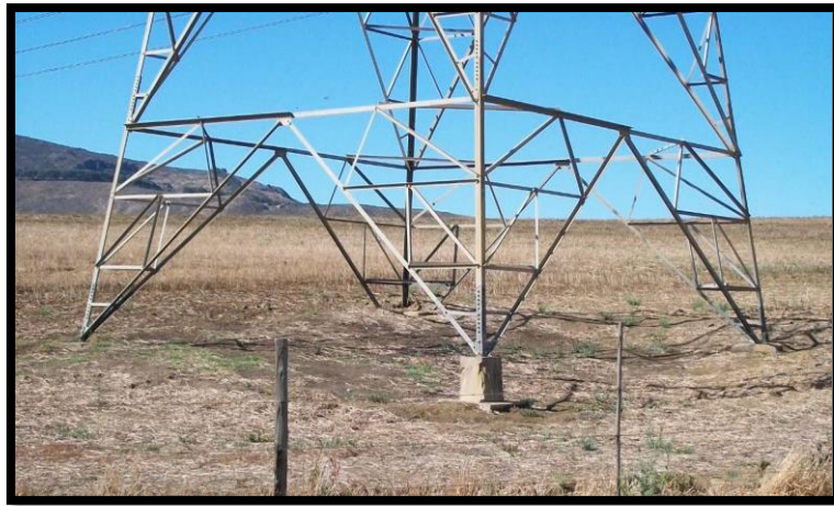
Photo 5.4: Typical dead man anchor foundations for guyed towers (Photo courtesy of Outeniqua Geotechnical Services, 2017).
