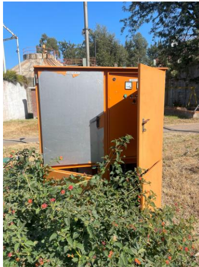
Figure: Decommission MCC and replace with new
