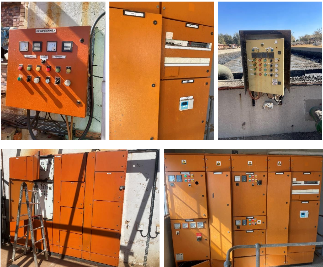
Figure: Refurbish Aerobic Digested Sludge Pump Station MCC & Decommission 3 x MCCs
