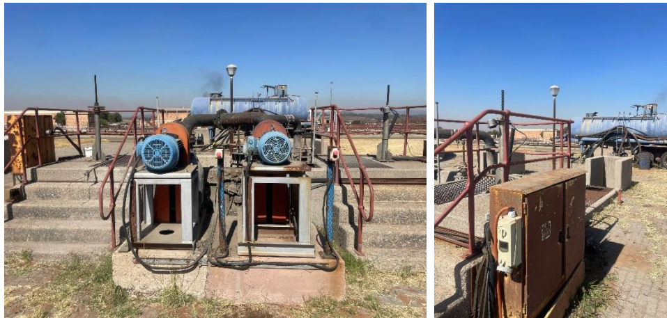
Figure: 2 x DBs & Industrial Welding Plugs to be Decommissioned and replaced with new
