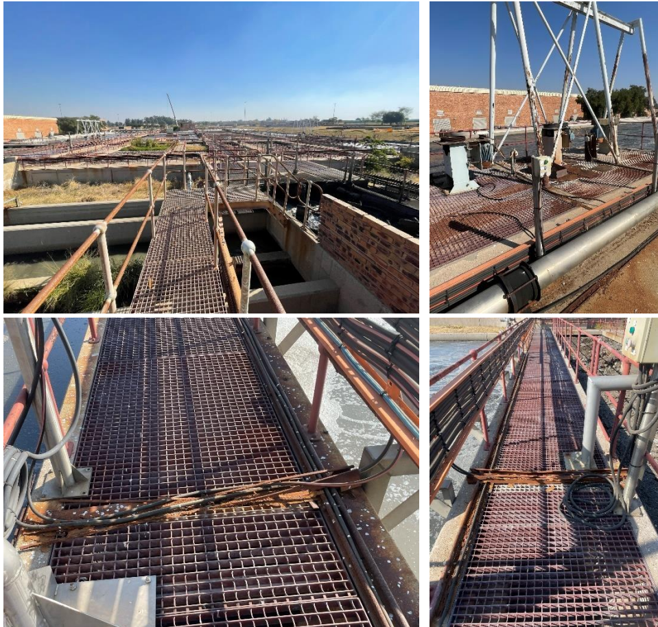
Figure: New power & control Cabling , racking and Aerial Lighting
