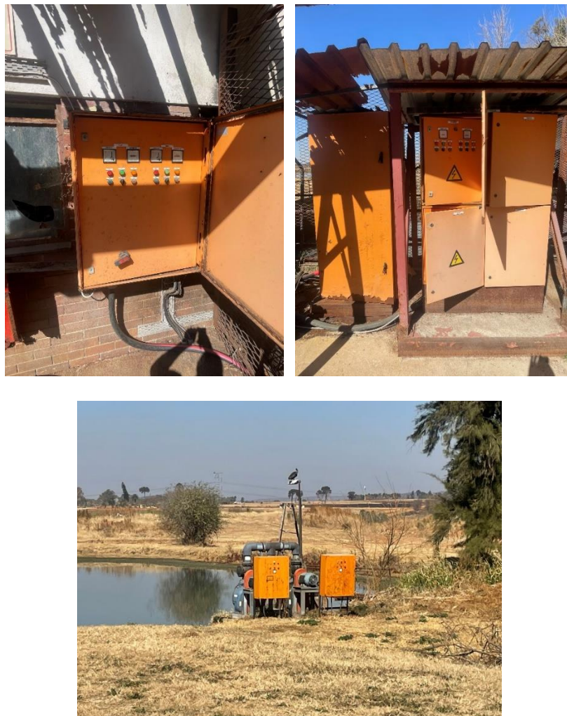
Figure: New MCC. Power & Control Cable Installation for all equipment & Decommission 5 x existing MCCs
