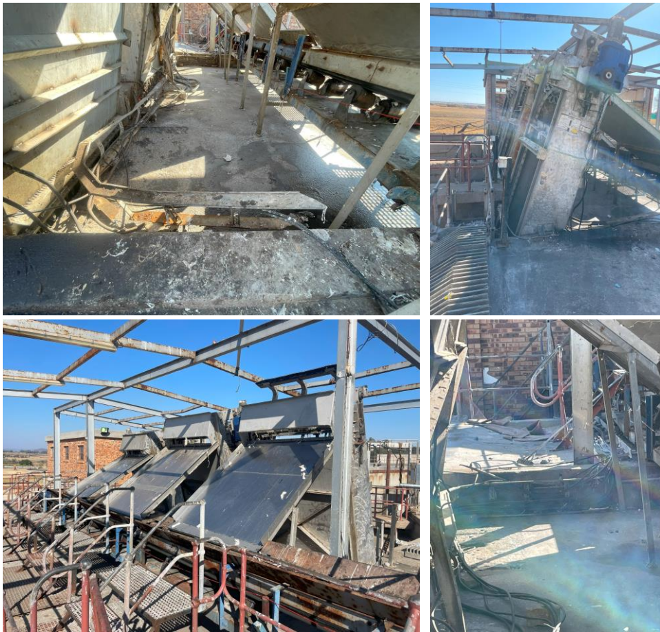
Figure: New power & control Cabling , racking and Aerial Lighting for Mechanical Screens.
