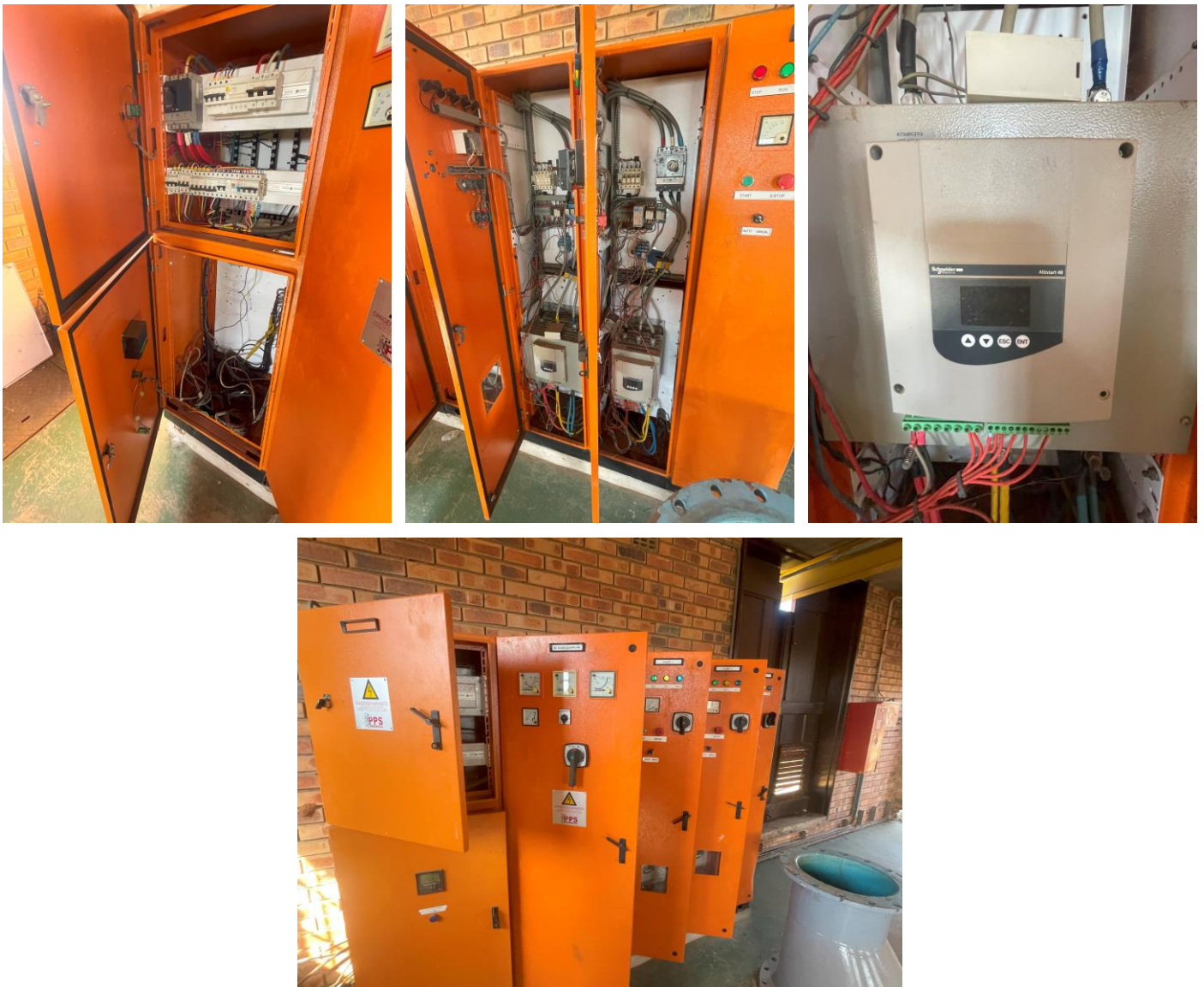
Figure: Refubish , Rewire & Install new Soft Stater in the Existing MCC
