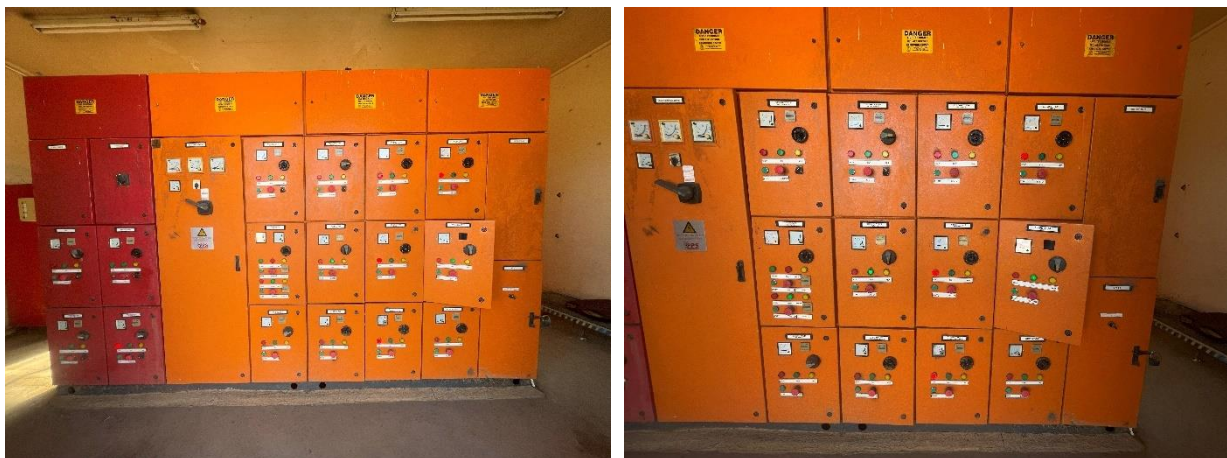
Figure: Existing Blower House MCC to be Refurbished.
