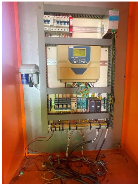
Figure: Reconfigure SCADA System and Installation of Power & Control Cables for new pumps (3 Off)
